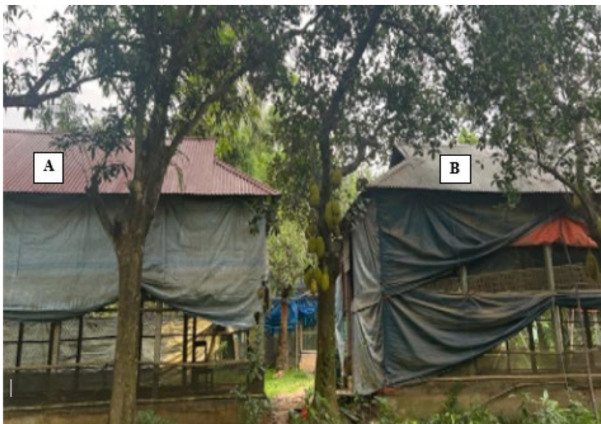
Figure 7. Coated with iron oxide primer (A) and uncoated (B).
